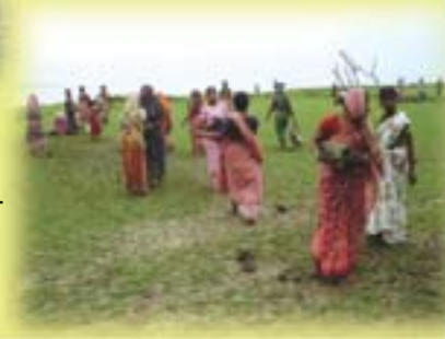
River embankment repairing by the villagers
